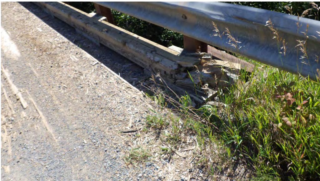
Photo 16: Impact damage at curb.
