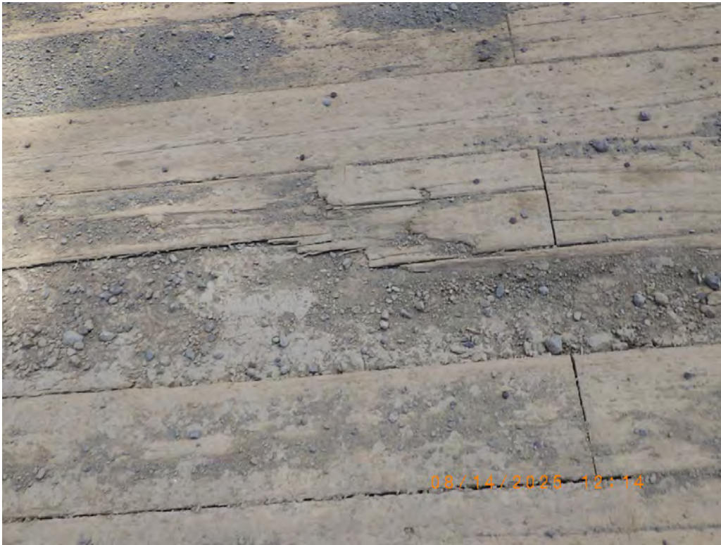
Photo 17: Severe rot at wearing surface planks.
