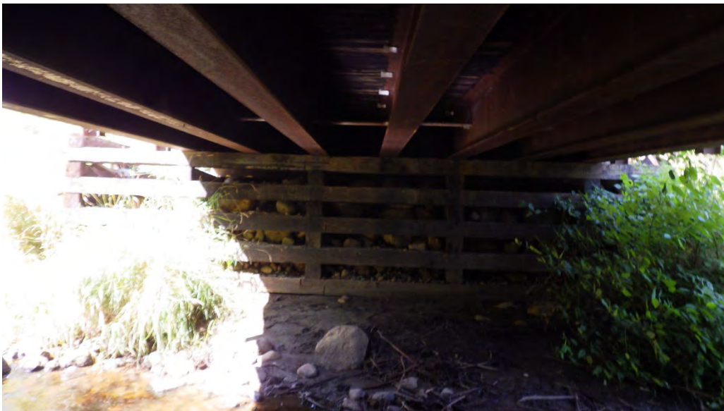
Photo 8: West abutment and embankment.
