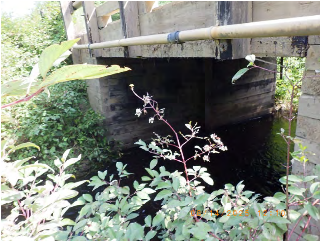
Photo 21: PVC pipe housing abandoned phone lines.
