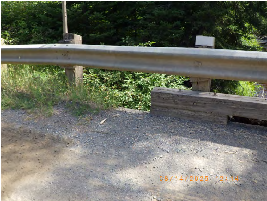
Photo 18: Curb does not extend full length of bridge, guide rail mounted 200 mm too high.
