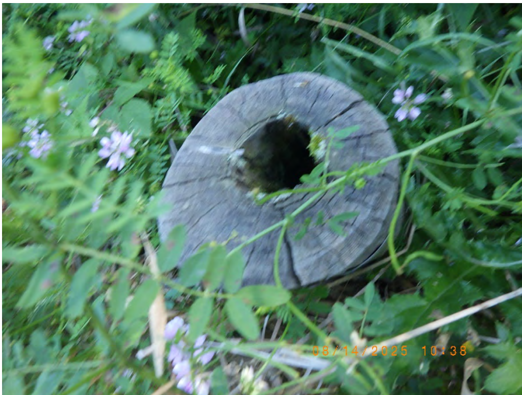
Photo 12: Severe section loss at guide rail posts.
