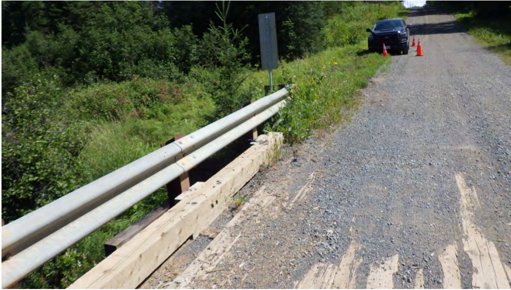
Photo 17: Gravel accumulation at corner of bridge.
