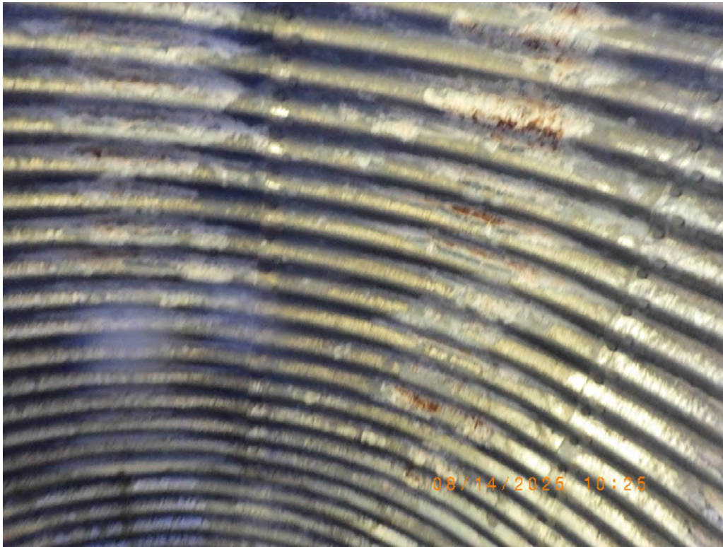
Photo 9: Light corrosion at top of barrel.
