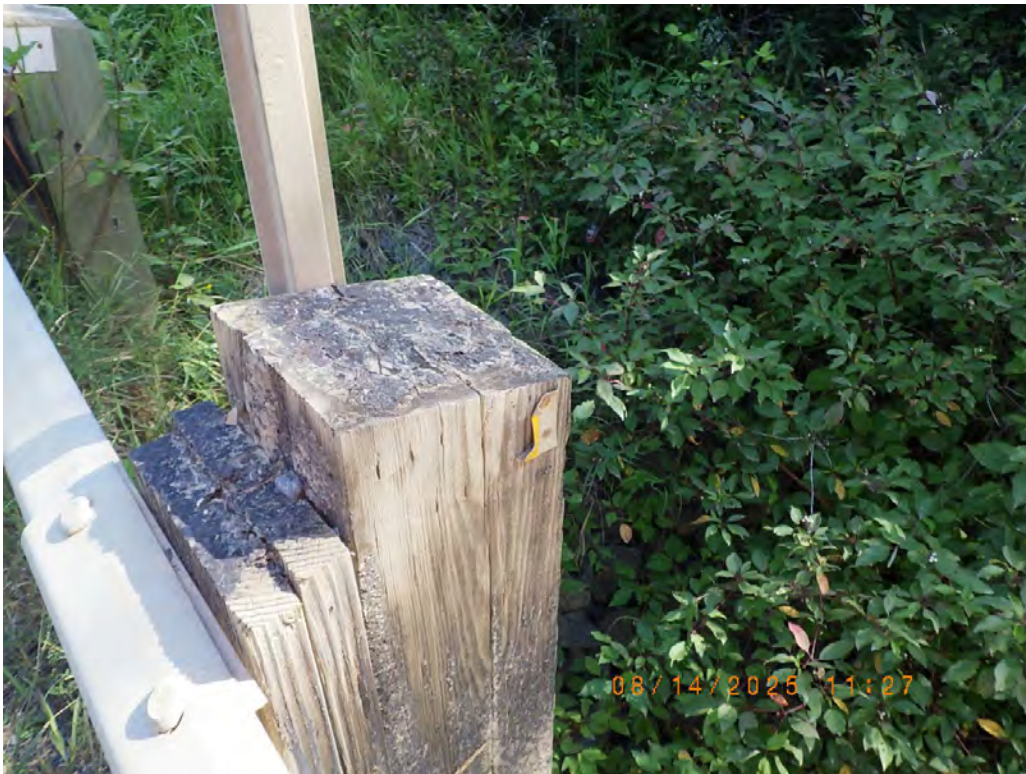
Photo 24: Broken reflector strip.
