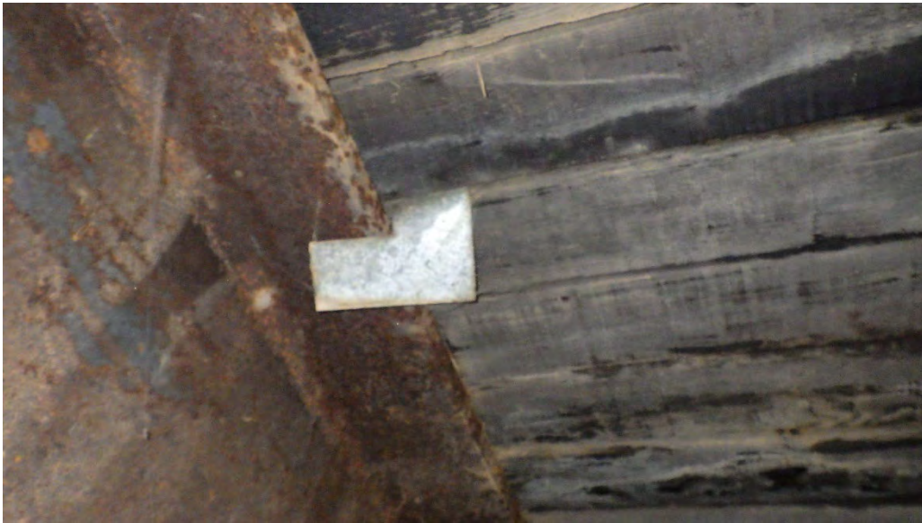
Photo 21: Damage deck clip (typ.).
