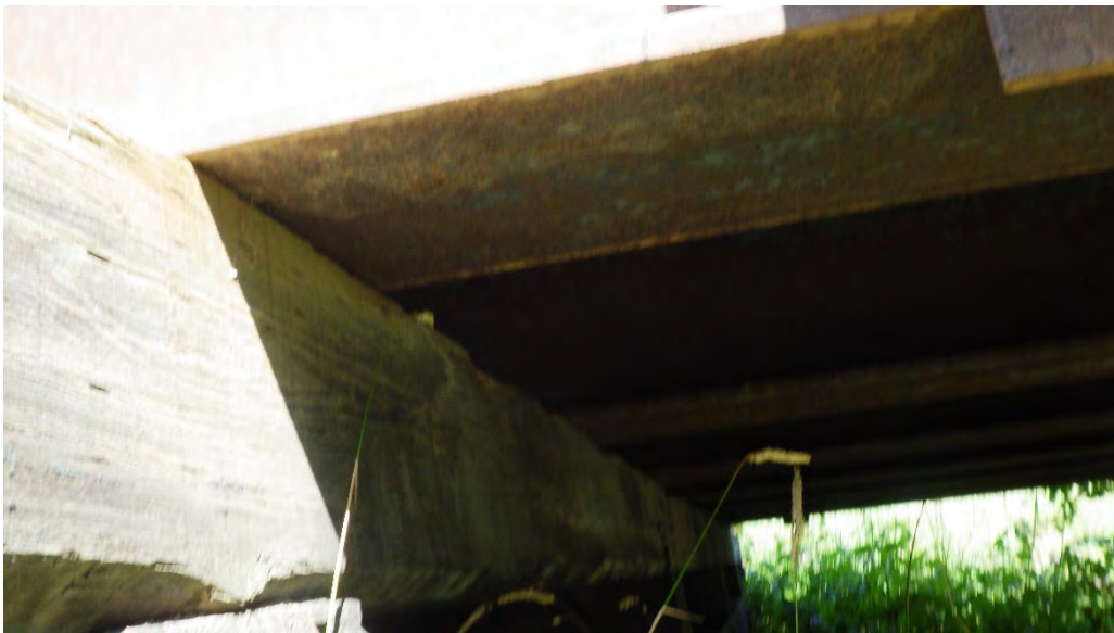
Photo 18: Girders bearing on front of abutment at west end.
