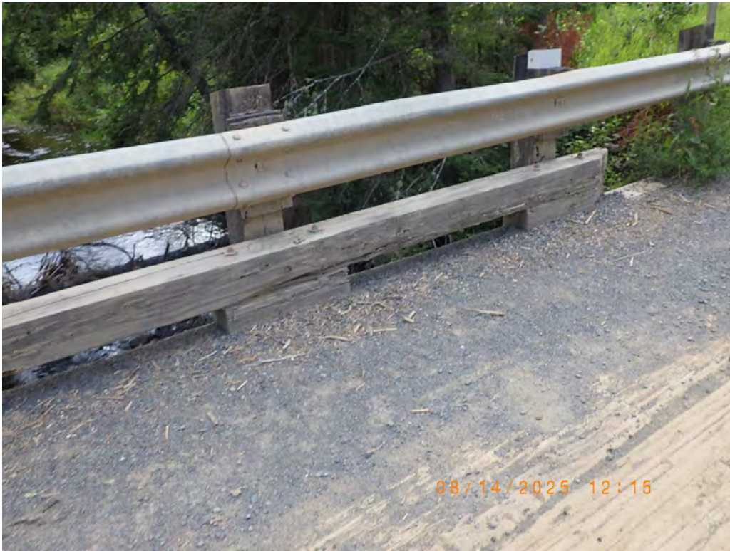
Photo 19: Medium abrasion at curb.
