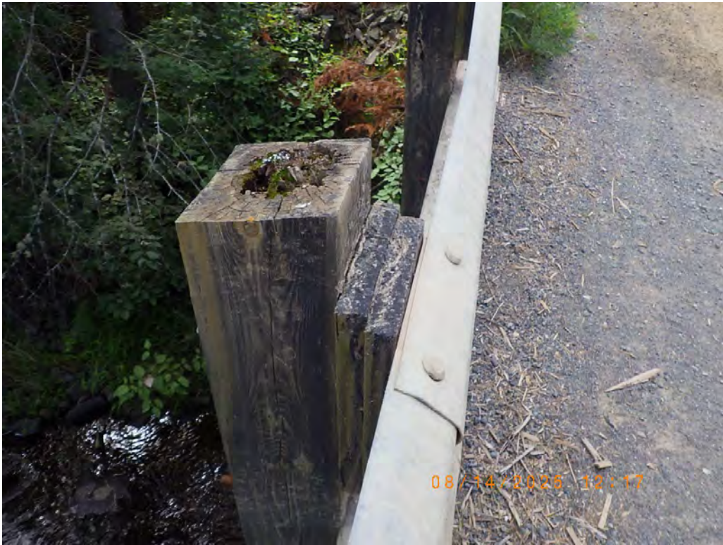
Photo 23: Medium to severe rot at posts.
