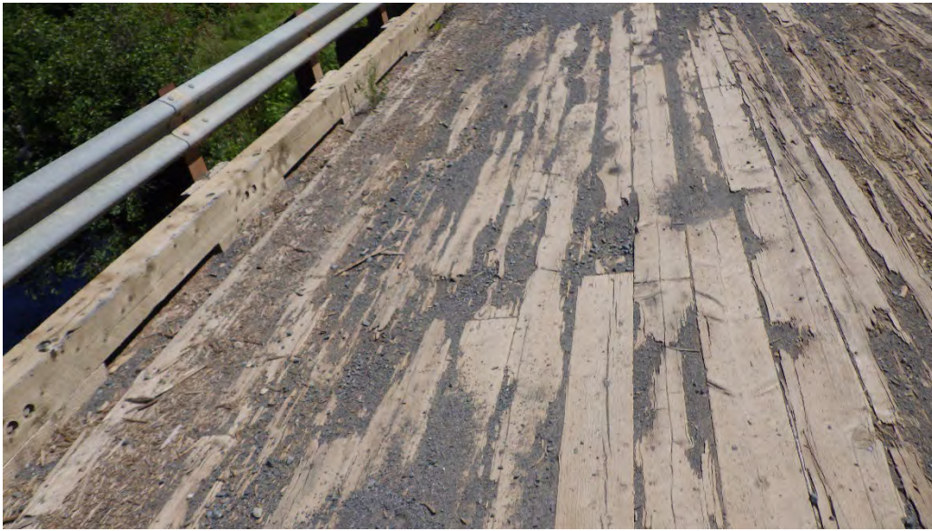
Photo 15: Severe rot at wearing surface planks.
