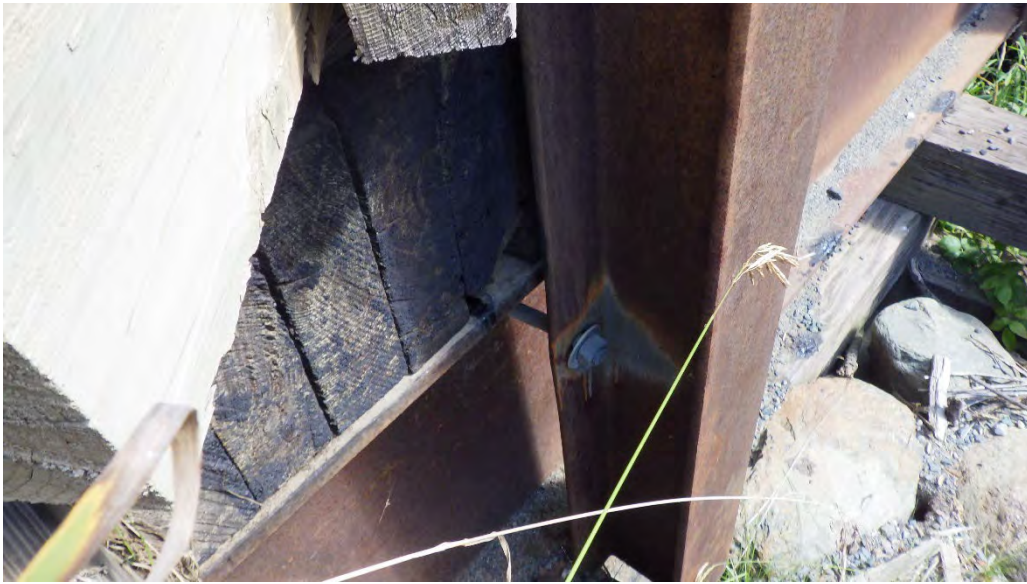
Photo 23: Loose bottom bolt on southwest steel post.
