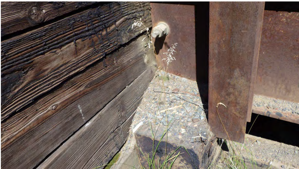
Photo 20: Gravel accumulation at bearing timber ends (typ.).
