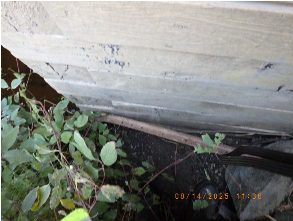
Photo 20: Loose steel angle next to southwest abutment.
