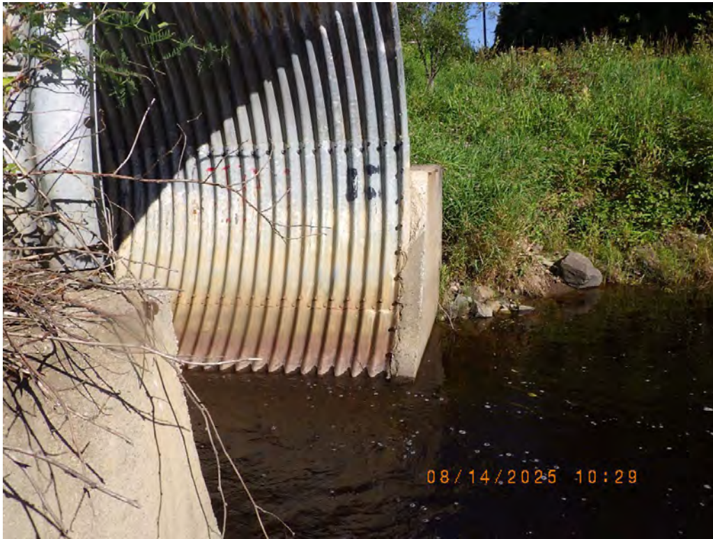
Photo 11: Scaling at downstream headwall.
