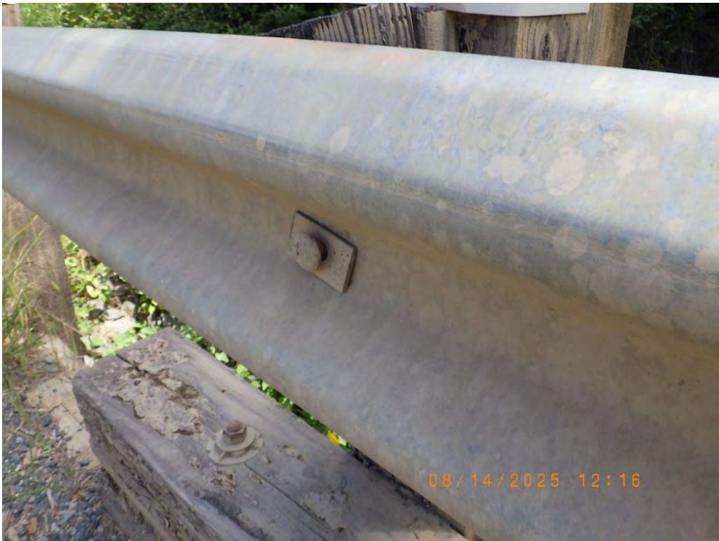
Photo 22: Loose guide rail splice bolt.
