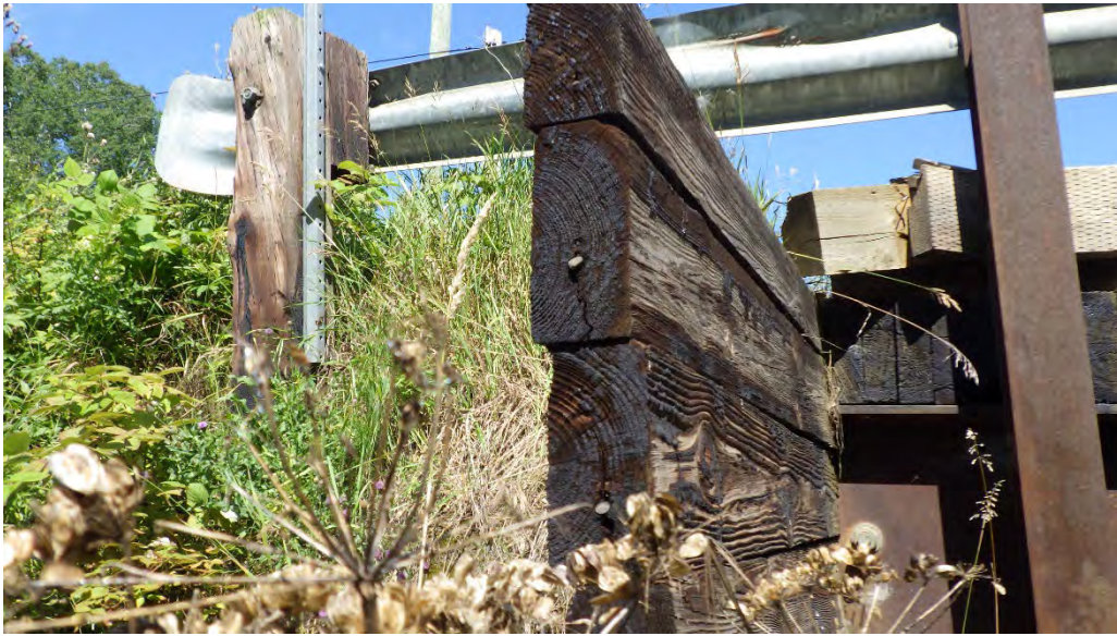
Photo 19: Crushing of ballast wall (typ.).
